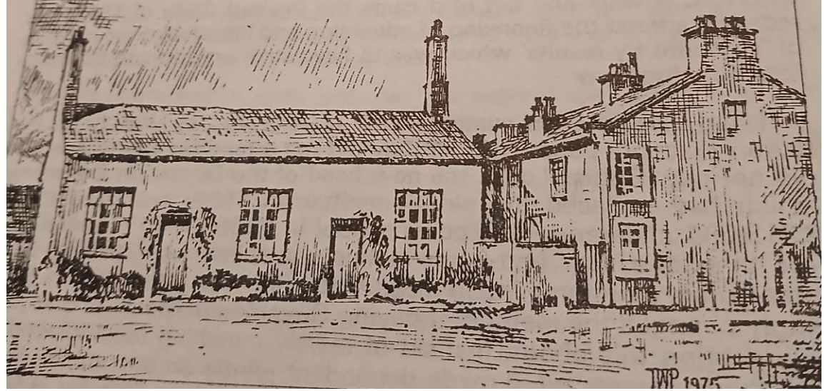
The second school in the square
